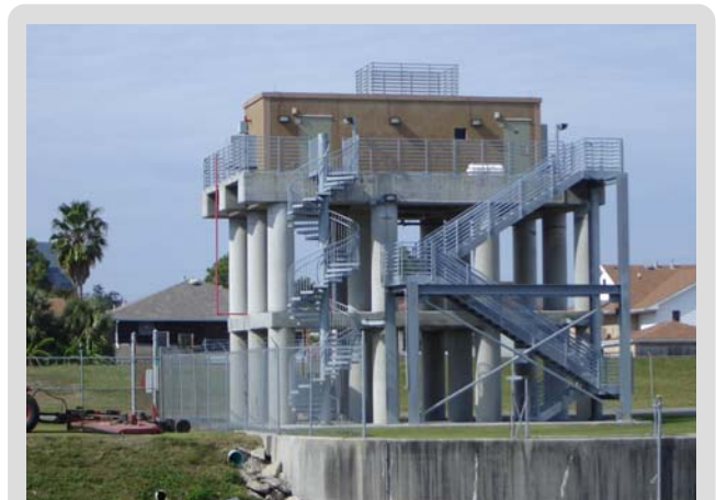
Safe house at Bonnabel pump station
