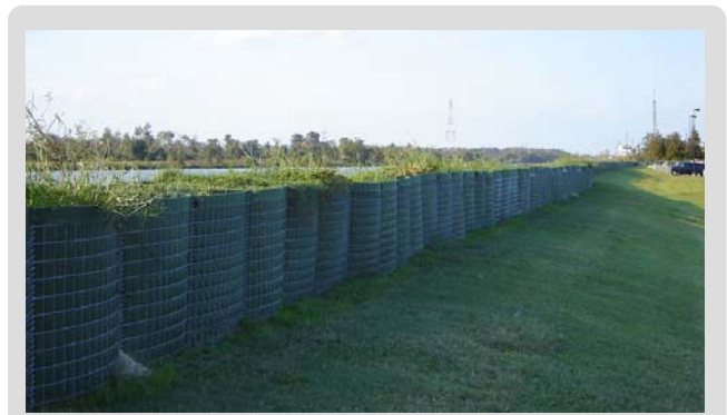
Interim flood protection along the Harvey Canal
