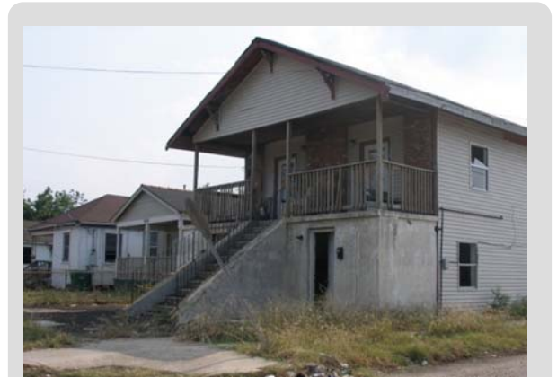
Flood related damages are covered by federally funded flood insurance policies, not by homeowner policies.
