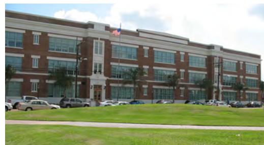
The school facilities master plan for New Orleans—completed in 2008—has guided decisions on school renovations and the construction of new school facilities.
