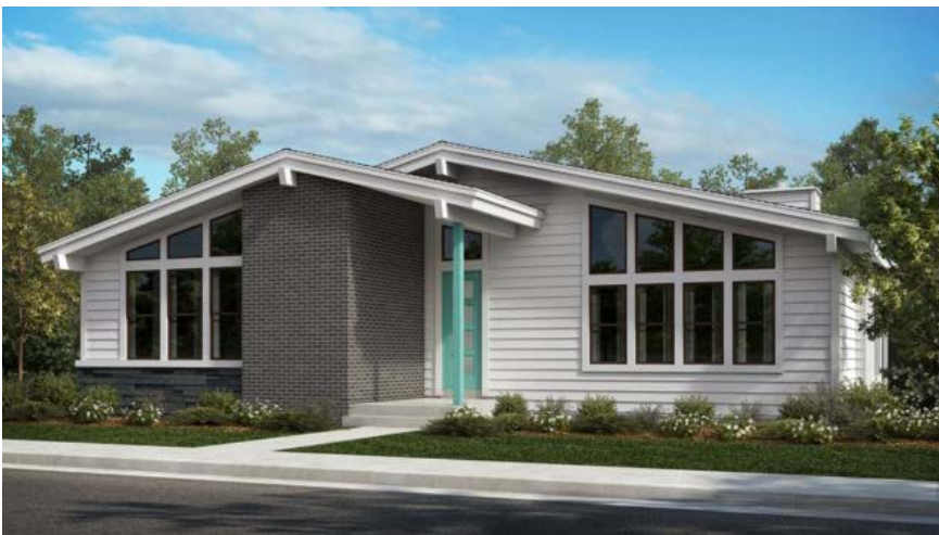
d. Same roofline pitch is extended to protruded area (front extension)
